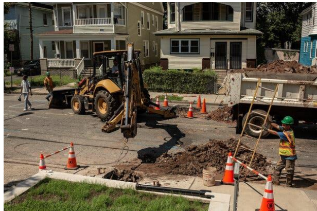
Workers removing lead pipes in Newark, N.J. $45 billion goes toward elimination of lead pipes. Credit - Bryan Anselm for The New York Times
